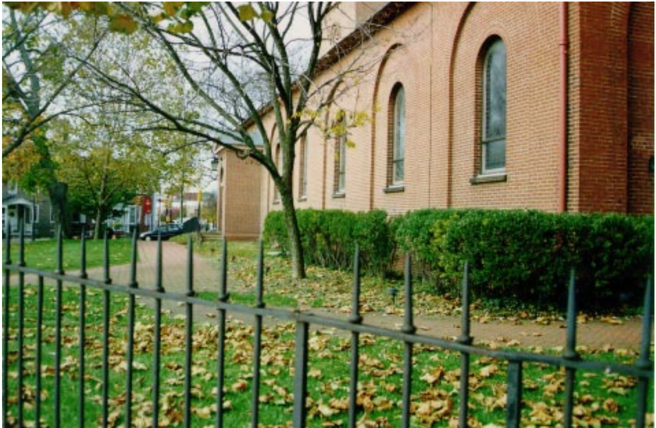
EXISTING BUILDING — VIEW FROM SIDEWALK, SOUTH
