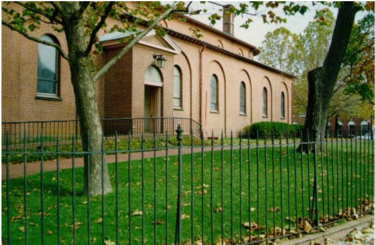
EXISTING BUILDING — VIEW FROM SIDEWALK, NORTH
