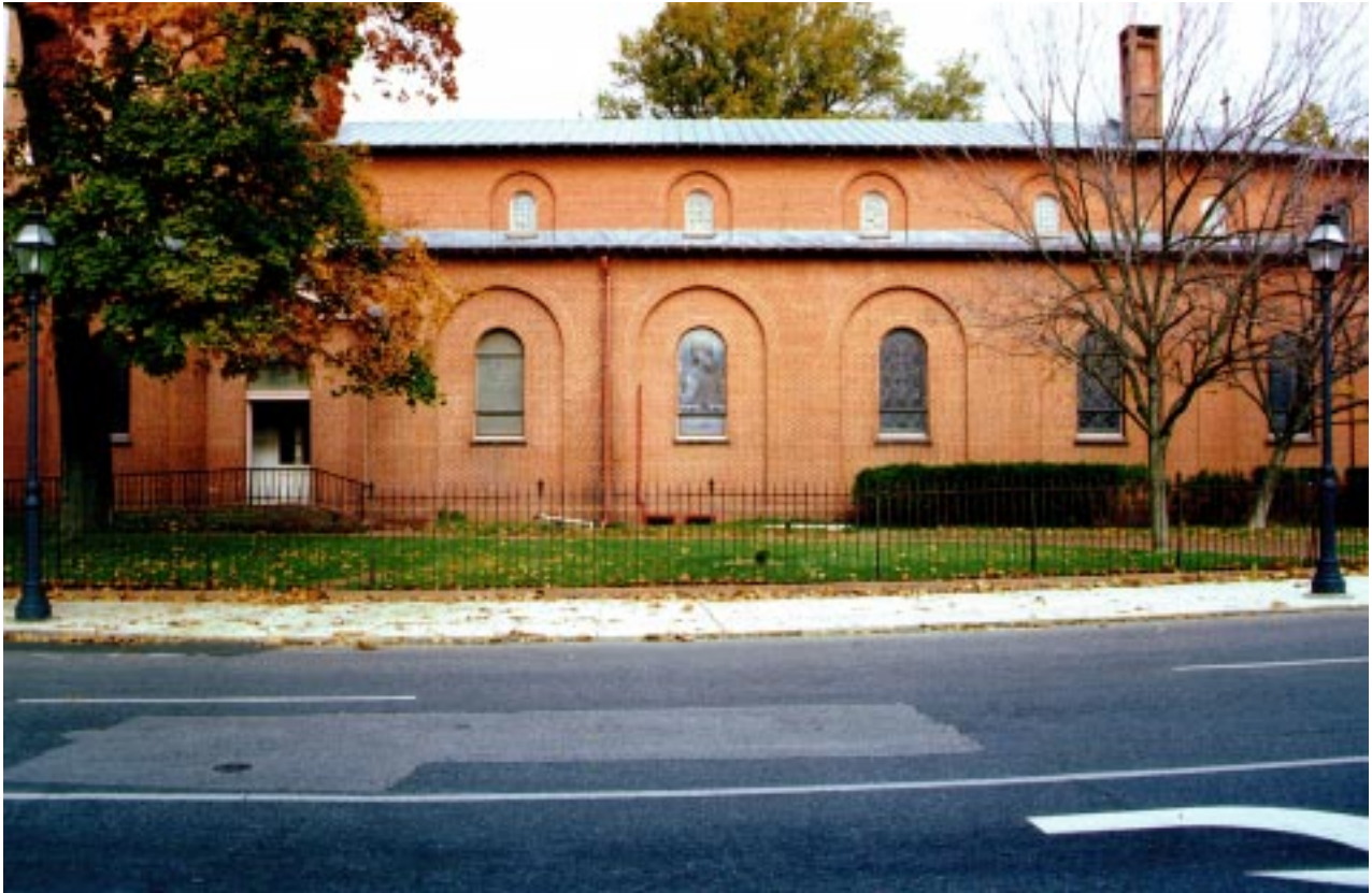
EXISTING BUILDING — VIEW FROM SIDEWALK, EAST
